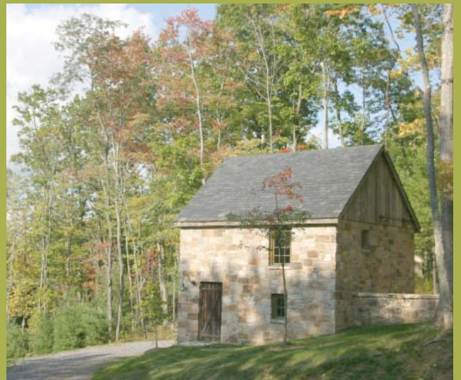
water pump booster station clad in stone with chestnut soffits and gable ends
