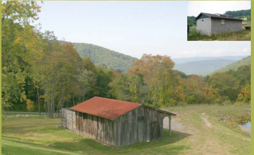
existing building clad in chestnut reclaimed from a nearby fallen barn
