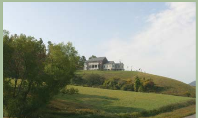
top: front elevation, bottom: muted colors and sited at edge of meadow minimize impact
