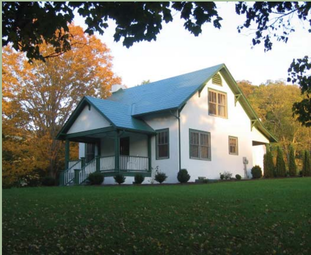
above right: barn, bottom right: main house, bottom left: views from front porch
