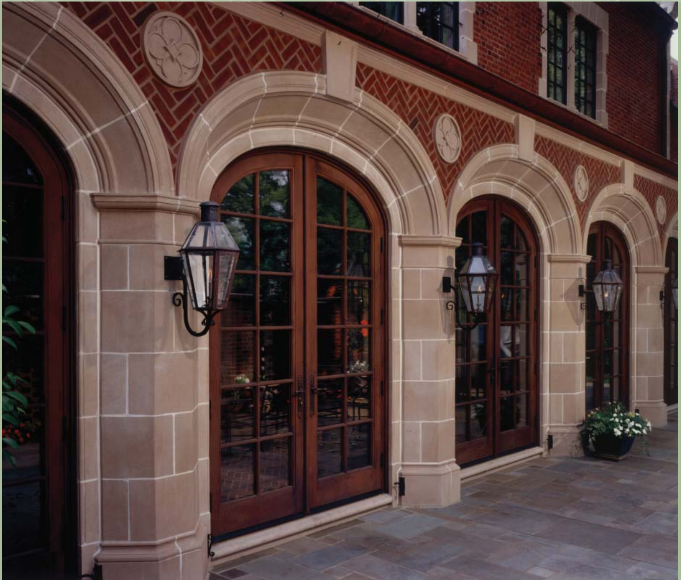
loggia at side garden
